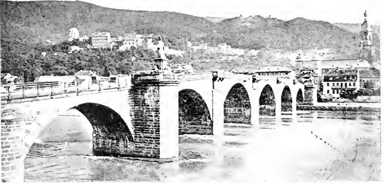
BRIDGE AT HEIDELBERG, GERMANY.
